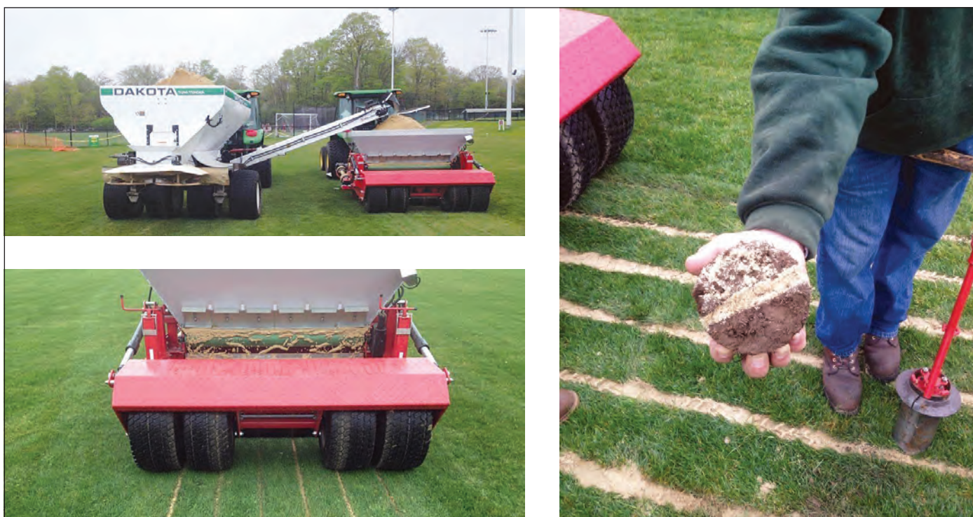
Sand-slit drainage system installation. Credit: B. Polimer.
