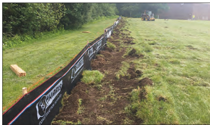
Sediment and erosion control measures. Credit: B. Polimer.
