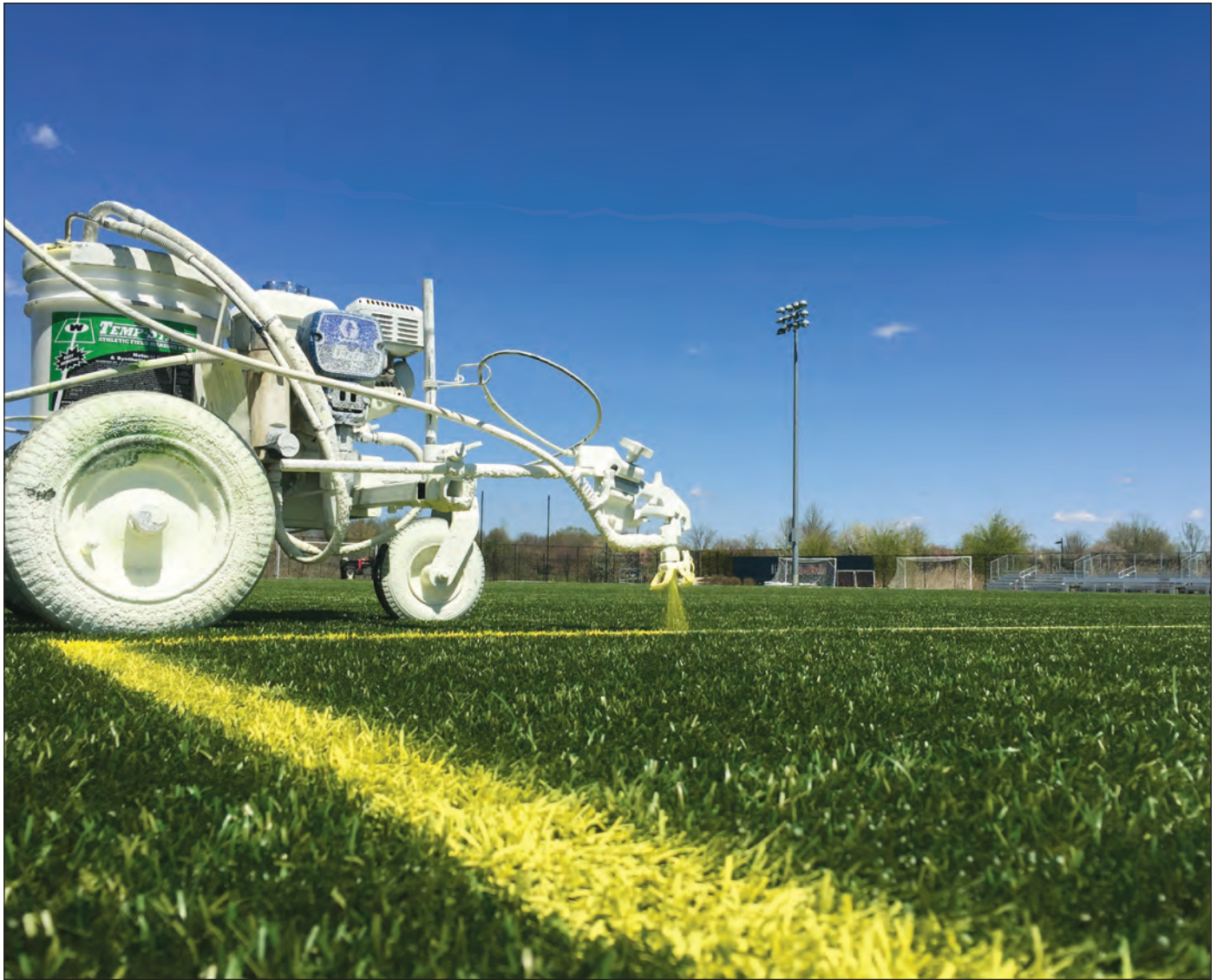
Paint application to sports field. Credit: Z. Holm.
