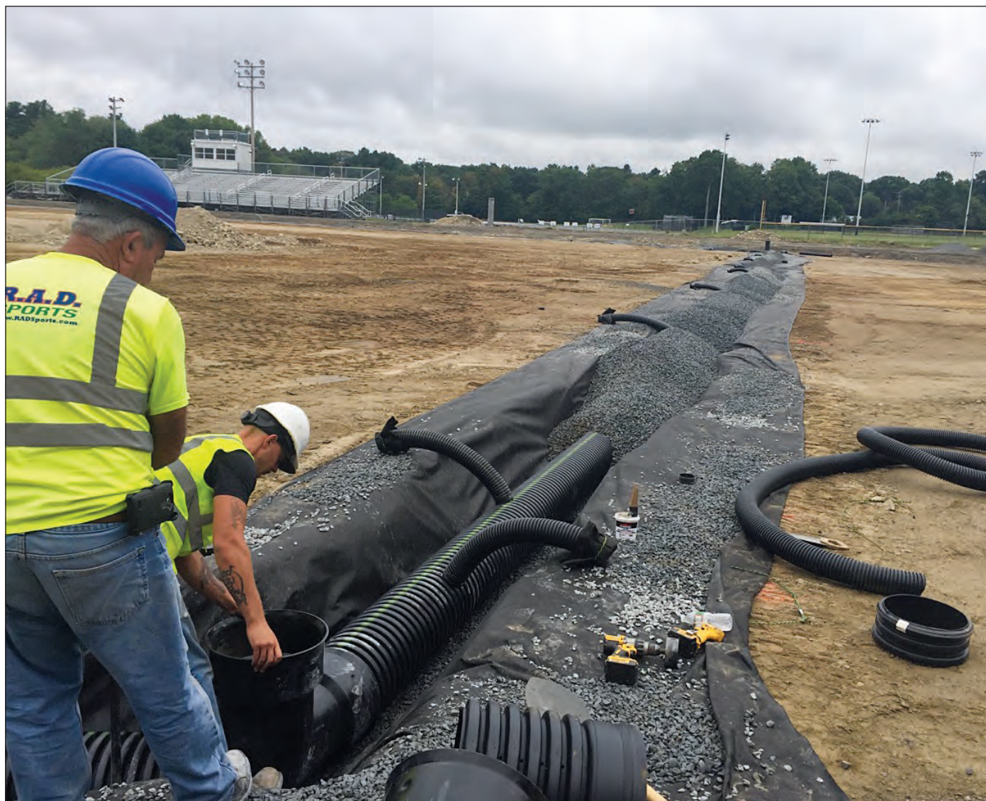
Installing curb drainage. Credit: B. Polimer.
