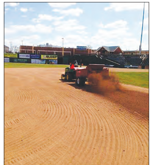
Application of infield mix. Credit: Z. Holm.
