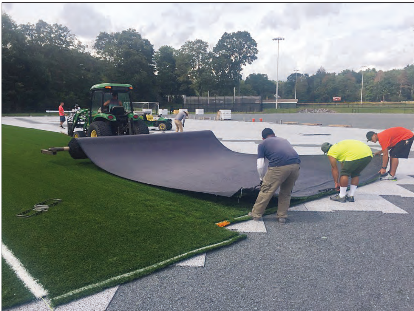
Synthetic turf installation. Credit: B. Polimer.
