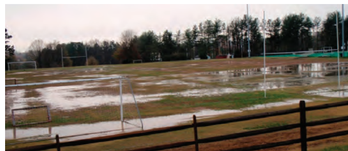
Standing water on an athletic surface - Photo courtesy of Chad Price, CSFM
